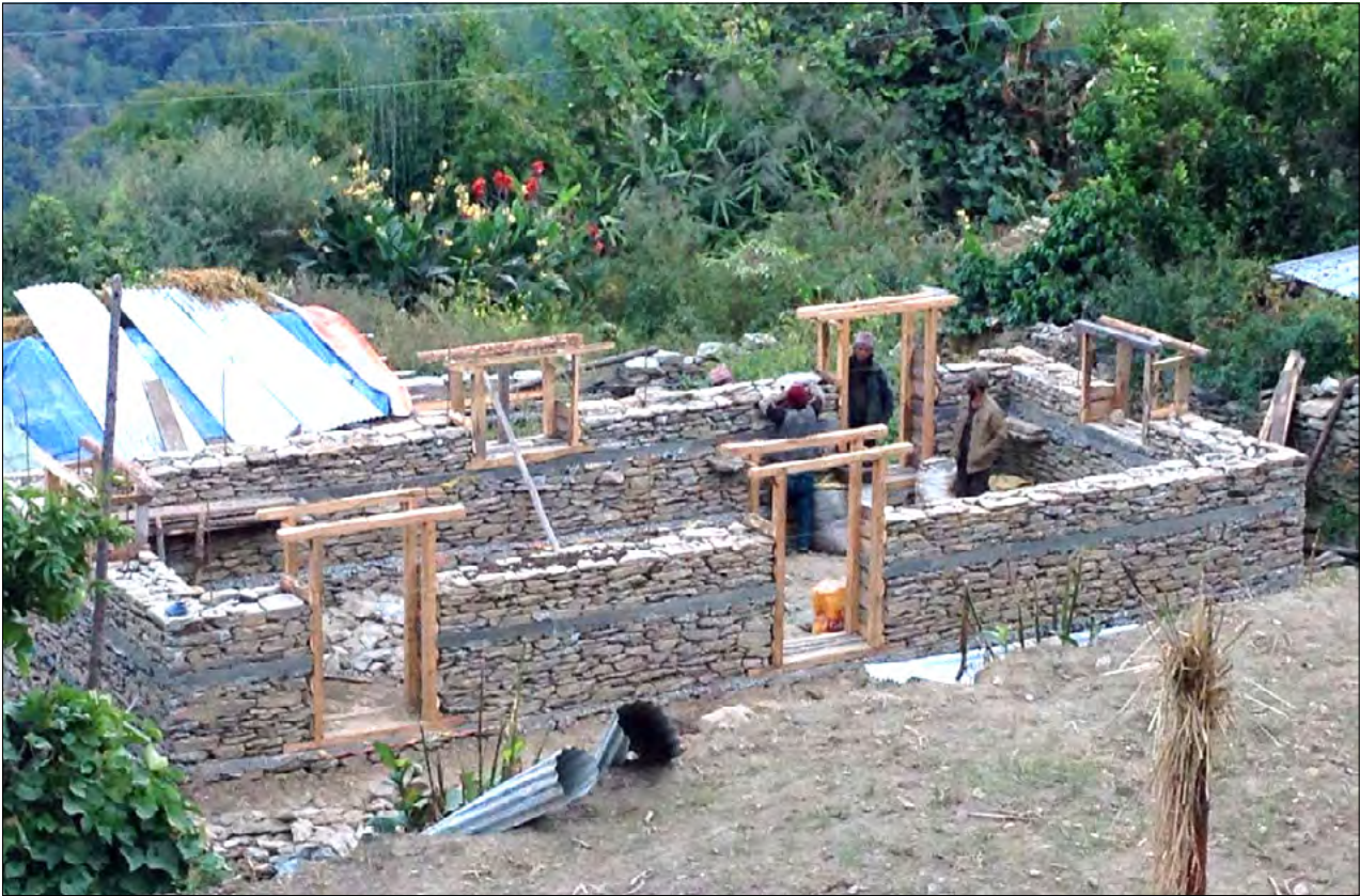
A house rebuilding in Dolakha—Photo: Chiran Manandhar
